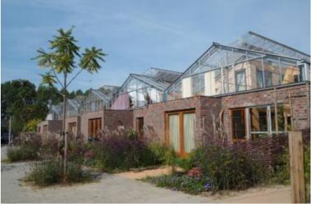
possible. The skeleton is made of wood and the walls of sandlime bricks The interior is also based on
